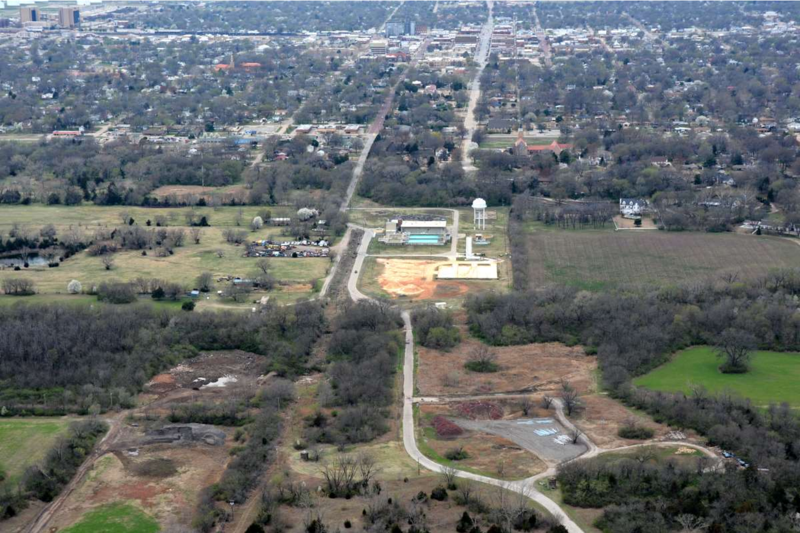
Top: Aerial photograph of Ponca, Okla. water treatment plant taken during the Oklahoma Wing Operations Evaluation, March 30, 2019. (Photo: Oklahoma Wing aircrew)
